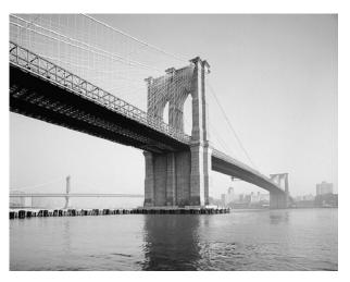
response of structures. This gives students an appreciation for the power of simple calculations as a tool for generating and validating new ideas, as well as the limited utility of complex, computer-based methods of analysis. Roebling's Brooklyn Bridge is an excellent example of an extremely complex bridge that was designed using only very simple methods of analysis.
